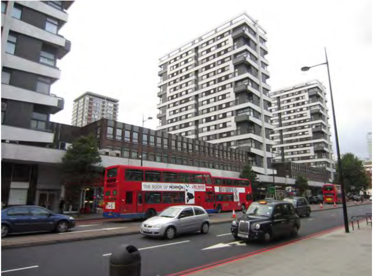
Front elevation from Edgware Road.
